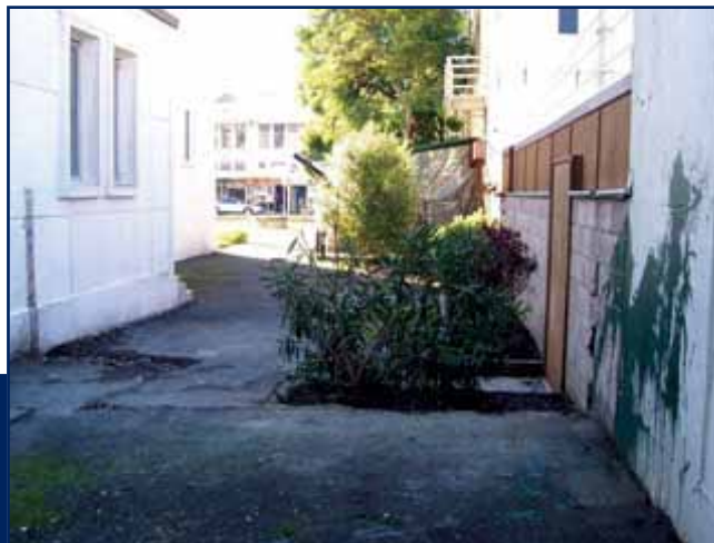
Two block walls completely removed. More lighting on right side. Clear view of both ends of the street.
