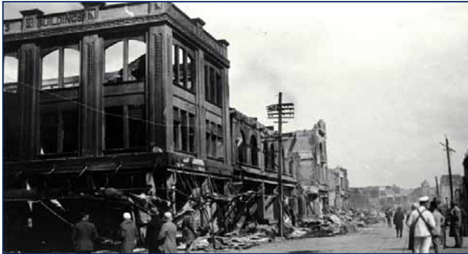
Napier Earthquake, 3 February 1931, Hastings Street.
